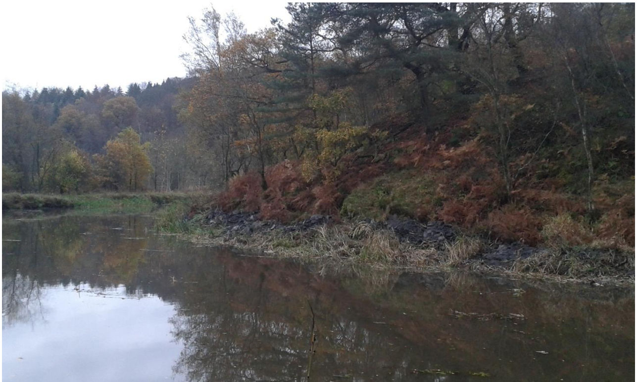
Above: Bankside disposal on offside bank at Strone Point on Forth & Clyde Canal
