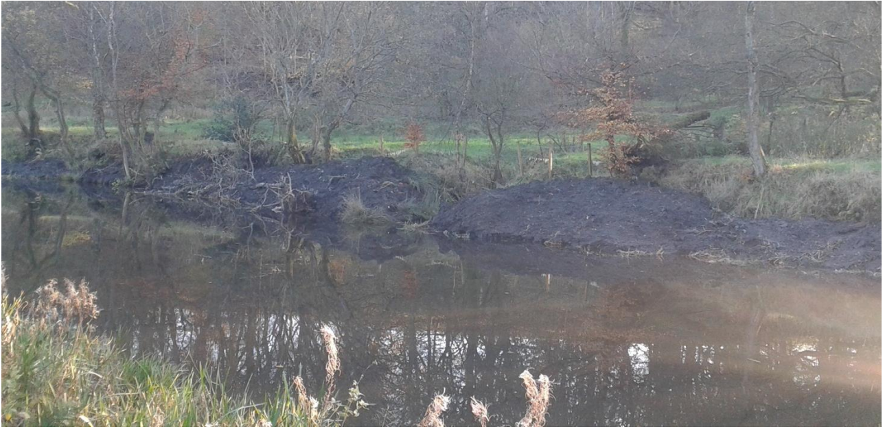
Above: bankside disposal on offside bank. Mound of material either side of burn entering canal on offside, clearly demonstrating where the burn deposits sediment underwater
