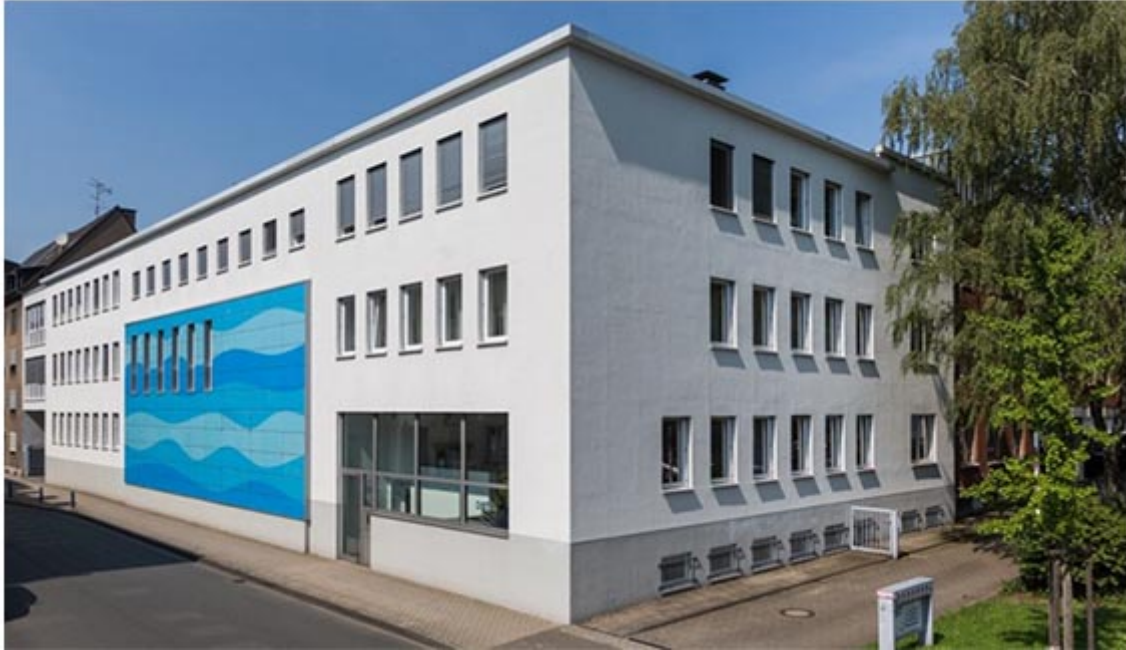
Figure 5: Development Centre for Ship Technology and Transport Systems in Duisburg, Germany, © DST
